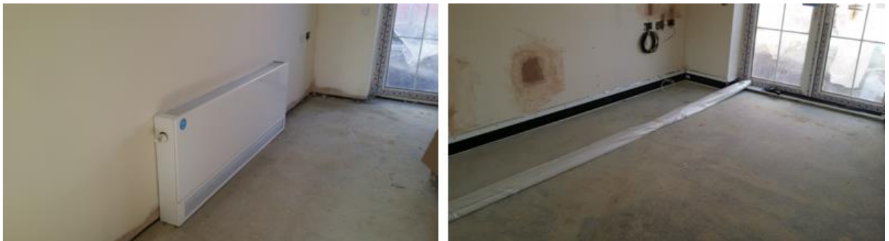
Even though the LST radiators had already been supplied, HB opted to swap them out for ThermaSkirt
