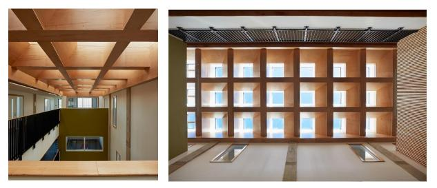
Pre-assembled to the GRP upstands, each rooflight was simply fixed directly to the concrete subconstruction. The single-ply membrane connection detail to the upstands meant that the roofing contractor was able to easily terminate the roofing membrane at the foot of the upstands. The upstands featured its seamless internal white construction, which therefore meant no dry-lining or decoration was required.
