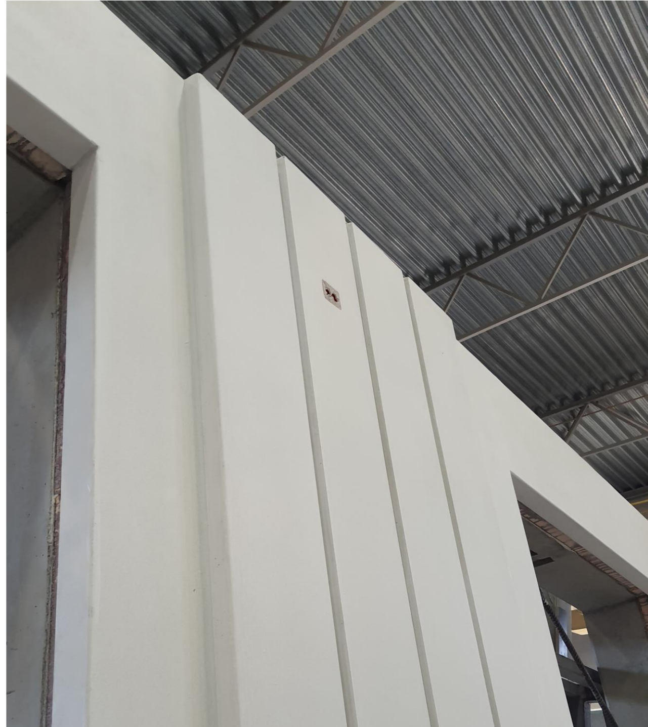
ELECTRICAL OUTLET in FACE PANEL
