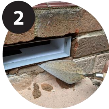
Mortar in channel
